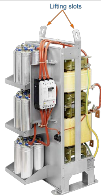
Figure 27 Location of lifting slots
