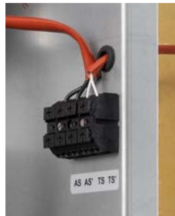
Figure 31 terminal for auxiliary contact connection
